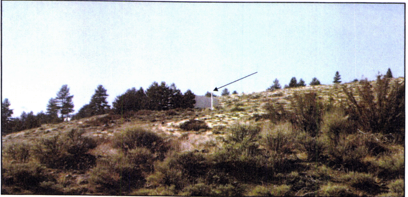
Photo taken from Timberline Drive with proposed monopole antenna facing west.
